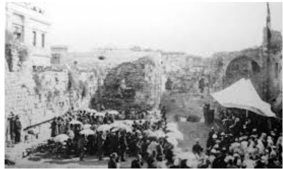
The foundation stone for the Church of the Redeemer was laid on October 31, 1893, in the ruins of St. Maria Latina. 74
